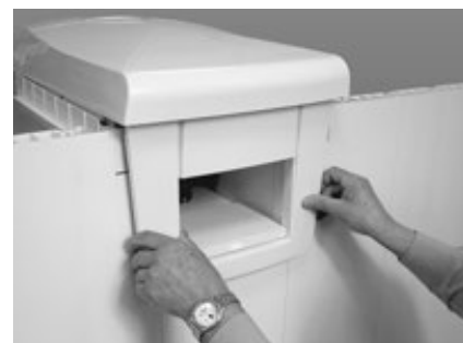
Put the trim with skimmer flap in position. Clip together.
